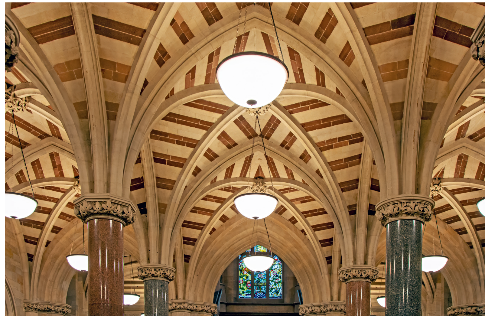
Ceiling of the Exchange on the ground floor
